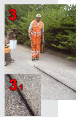
Heat the compound slowly in a melting pot equipped with a stirrer and a thermostat to the working temperature of approx. 160°C. Caution: Overheating (over 180°C) will destroy the compound!
