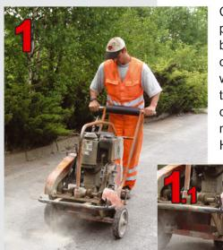
Cut the joint wide enough for pouring (max. 2cm) (Fig.1). Then blast clean the cut joint with compressed air (Fig. 2) or clean with a brush machine. To assure the required adhesion of the compound, the sides of the joint must be primed with BORNIT®-Haftgrund (Fig. 3).
