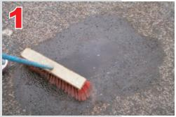
The asphalt pavement is cleaned with a broom of any standing water or soilage.
