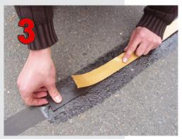
BORNIT-Crack Tape must be lay out (picture 3) and pressed on the crack area by roller, car tire or pounder (picture 4).
